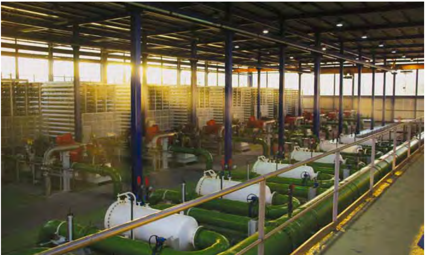
Inside the second largest desalination plant in the world, located in Torrevieja, Spain, and built under a 15-year design-build-operate contract by Acciona Agua. The plant delivers 240ML/d to the populace around Alicante, Spain.
