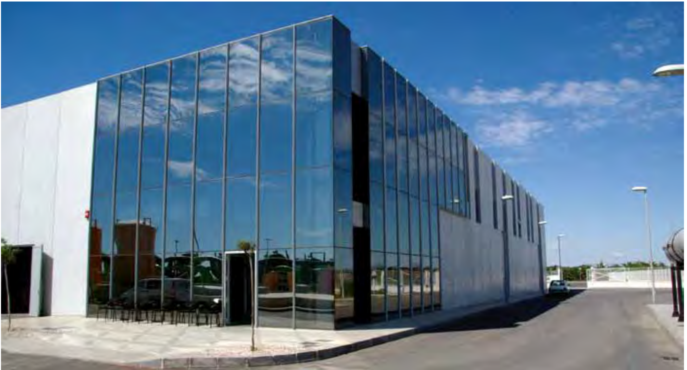
Cartagena II is one of two 65ML/d seawater reverse osmosis plants in Murcia, Spain, built on a 15-year design-build-finance-operate basis. The phase I plant was constructed by a consortium of Acciona Agua and Befesa. Phase II was constructed by a consortium of Acciona Agua and Degrémont.
