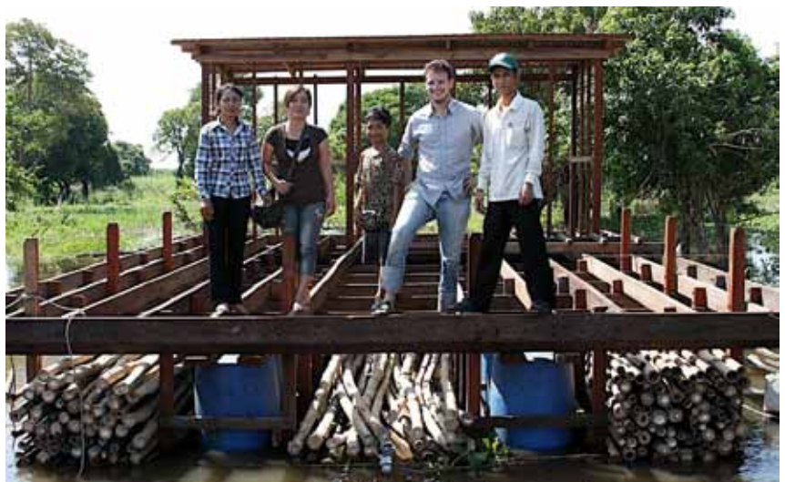
The project team with the Community Waste Management Station, a floating waste treatment barge, under construction.
