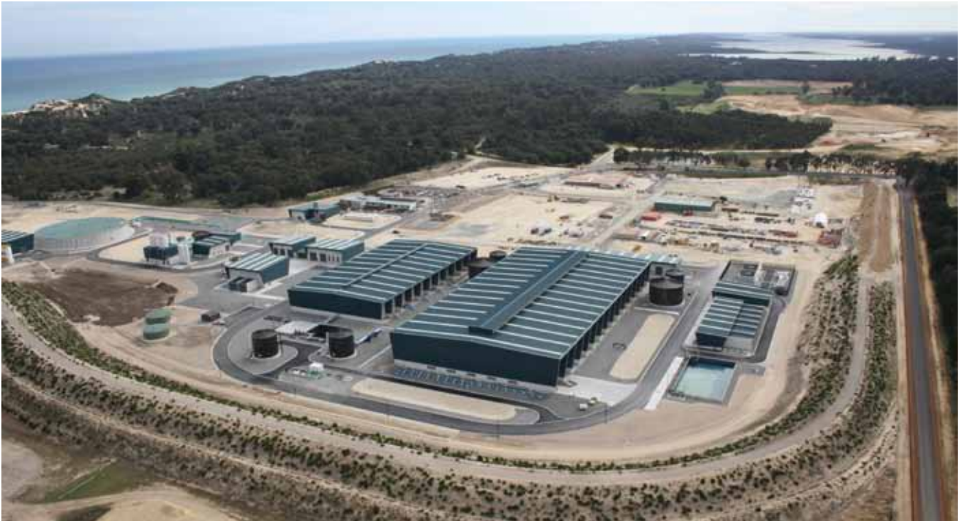
Perth's second desalination facility, the Southern Seawater Desalination Plant, has started operating and is planned to reach capacity of 100GL/a.
