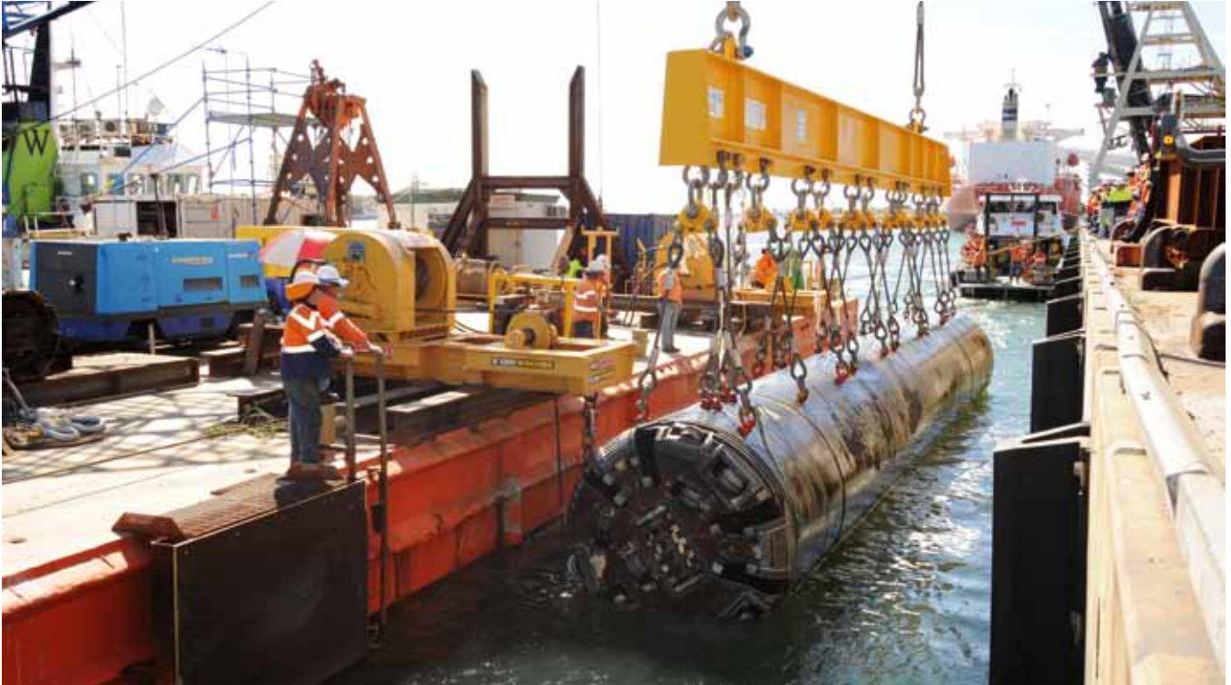
Recovering a TBM from the seabed.
